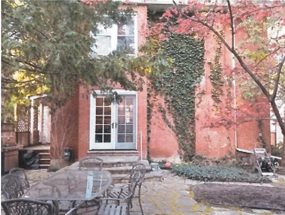
Existing backyard, looking east
