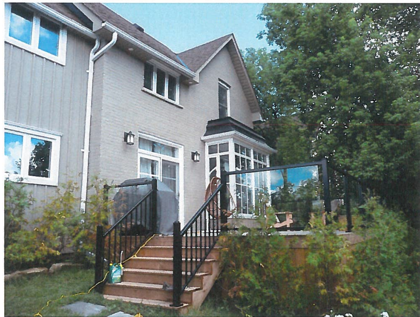
View of Existing Porch, looking North
