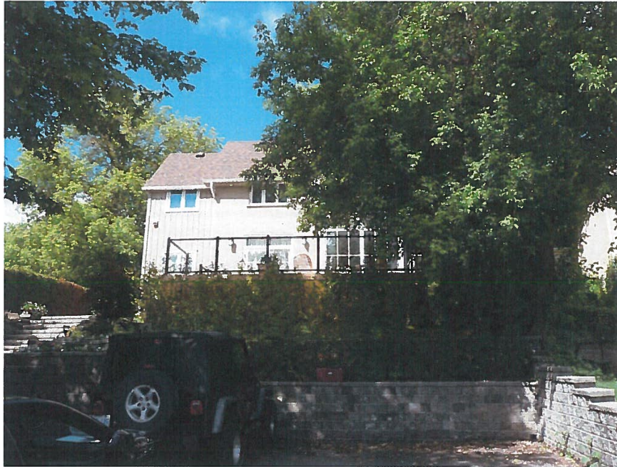
Front Elevation from Mill Street
