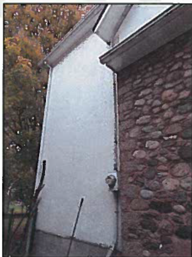
Figure 9: Right and Below: West wall showing edge of two storey north addition and recladding plus a change in the window of west roof gable, 2016
