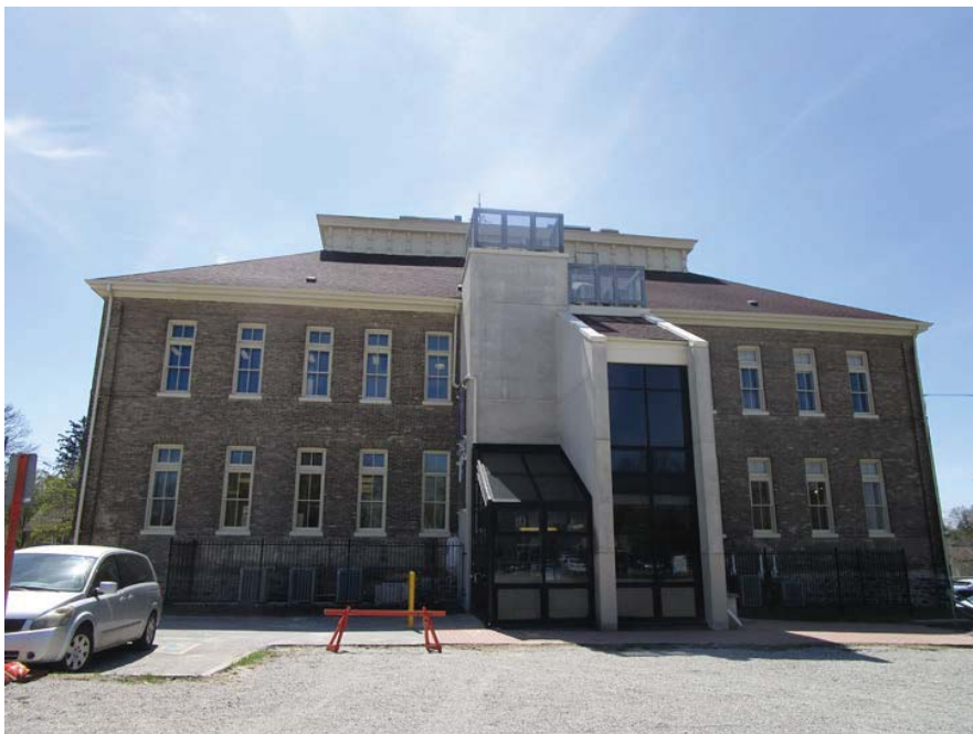
North elevation of 22 Church Street (ERA, 2018).
