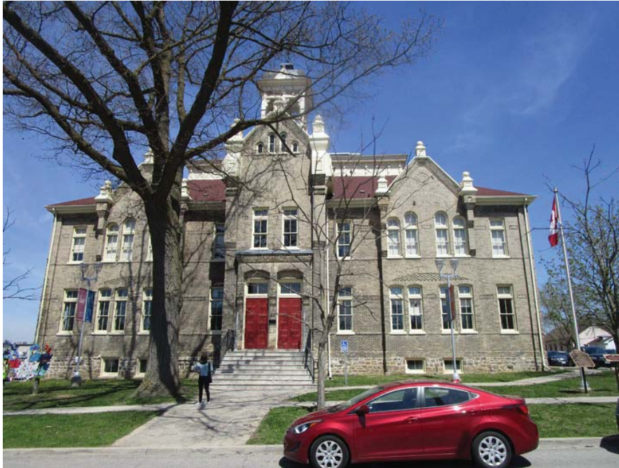
South elevation of 22 Church Street (ERA, 2018).
