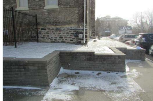
Detail of stone foundation and basement window at west elevation (ERA, 2019).
