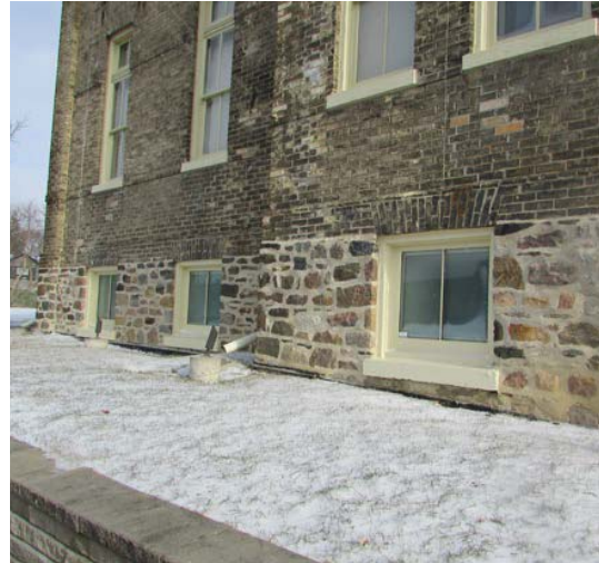
Foundation and basement windows at west elevation (ERA, 2019).
