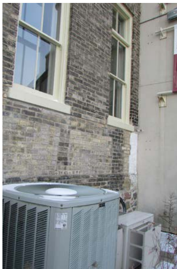
Detail of brick at north elevation (ERA, 2019).
