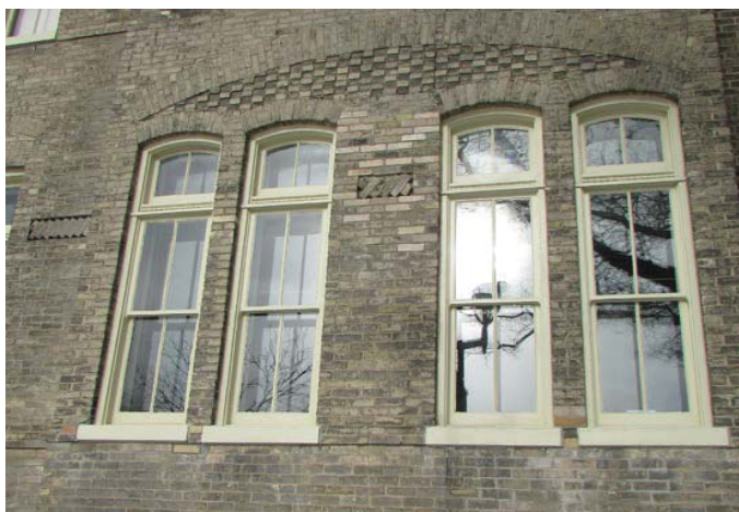
Windows at the south elevation (ERA, 2019).
