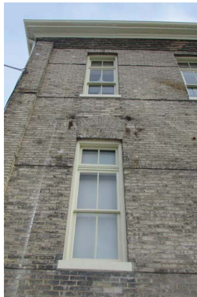
Ghosting on brick from removed fire escape stairs at west elevation (ERA, 2019).
