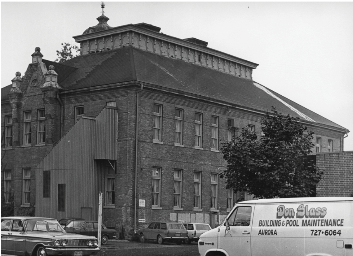
Southwest view of the school showing fire escape at east elevation, date unknown (Aurora Archives).
