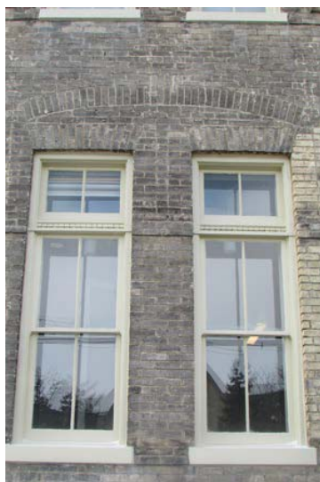
Windows at east elevation (ERA, 2019).
