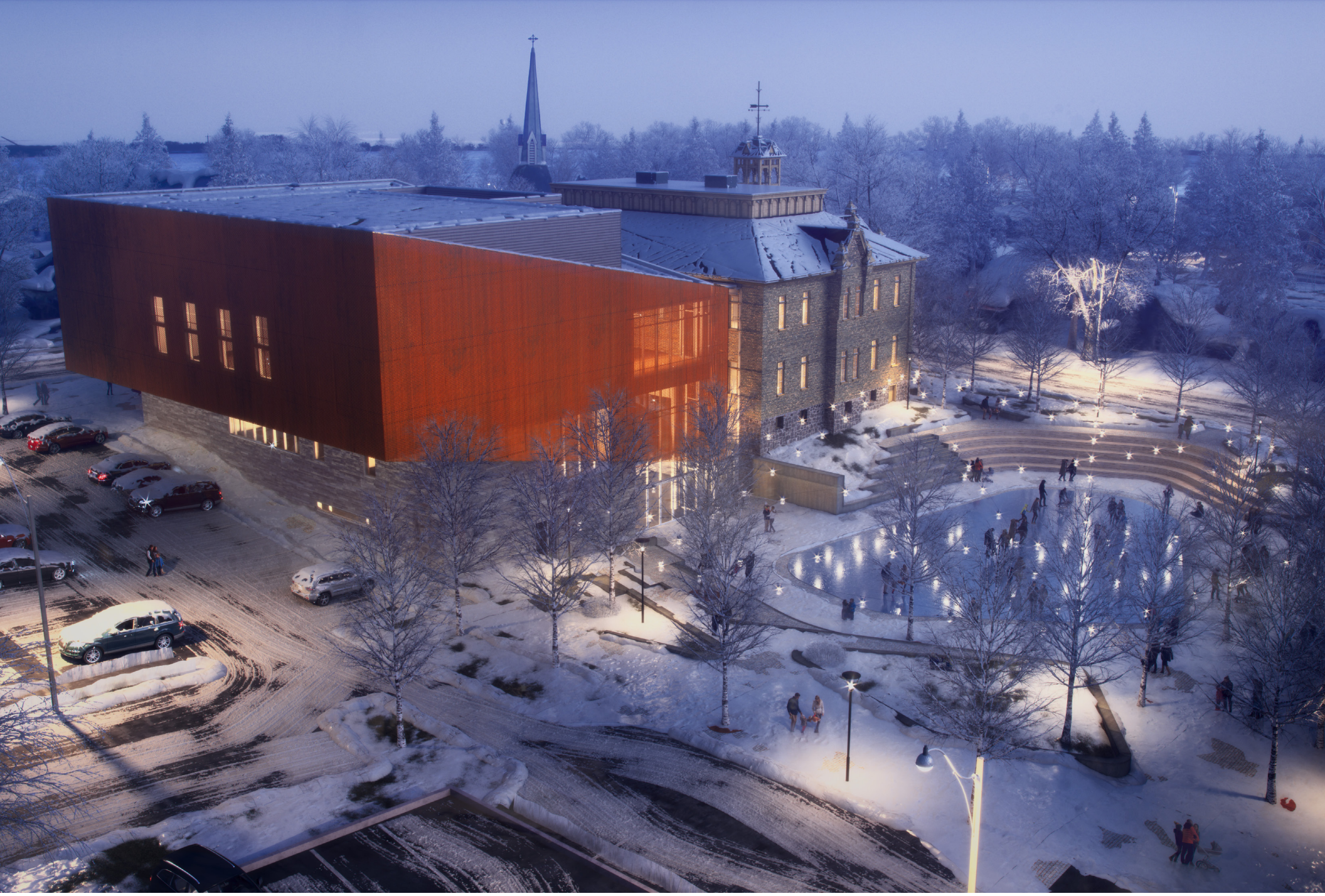
VIEW FROM CHURCH STREET
