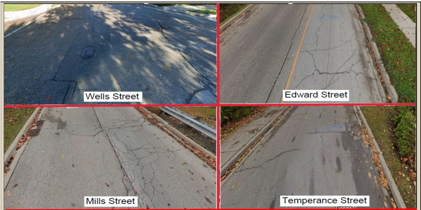
Figure 2: Site Photos Showing Existing Pavement Conditions
